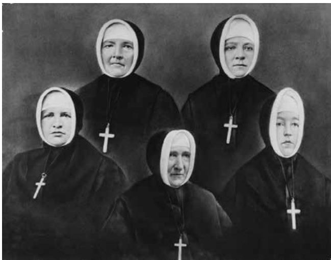
Top Row: Sister Vincent de Paul and Sister Mary of the Precious Blood. Bottom Row: Sister Praxedes of Providence, Mother Joseph of the Sacred Heart, Sister Blandine of the Holy Angels. Sisters of Providence Archives.
