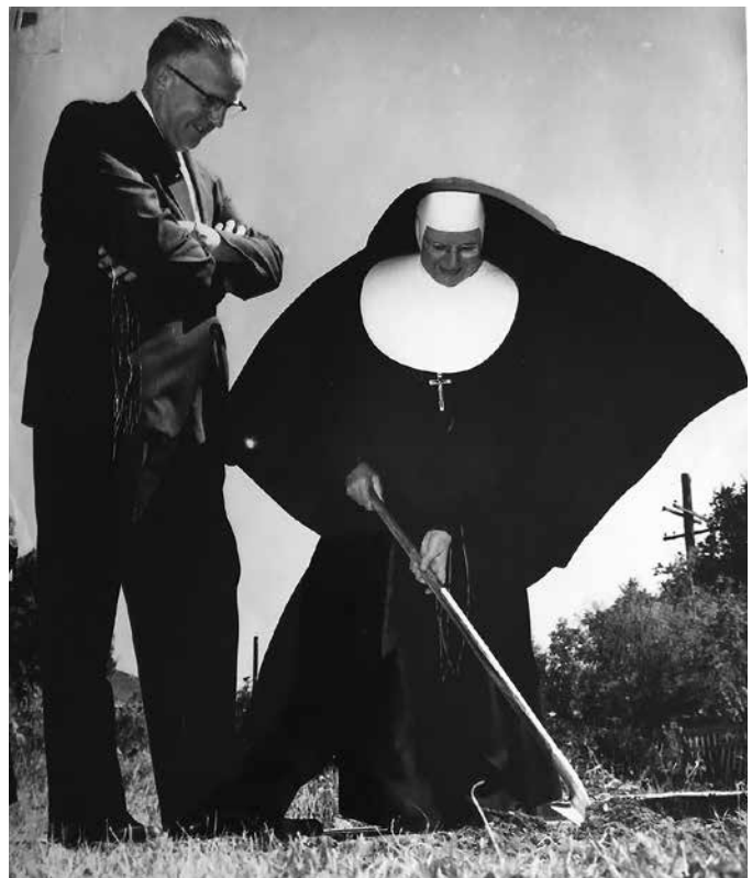
Dr. Ralph Christenson and Sister Theodore Marie Gorman break ground for the School of Nursing building, Eugene, 1964. CSJP Archives.
